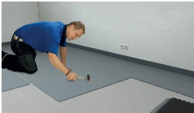
Tip: Laying with a soft-face hammer
